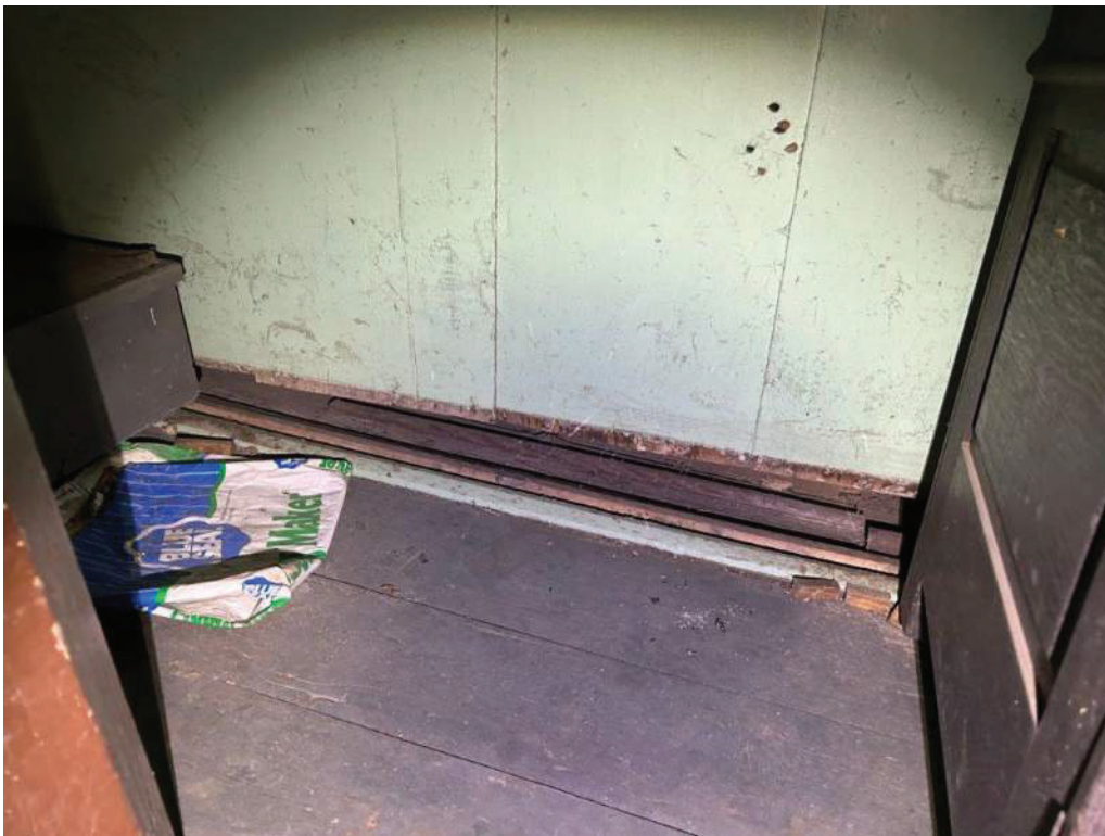
Photo 16 Drop in basement floor
