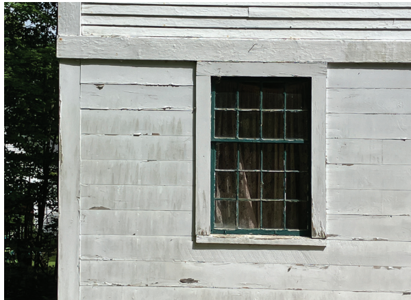
Image A-27: Lower level windows are “cottage style”, or double-hung with top sash shorter than the bottom sash
