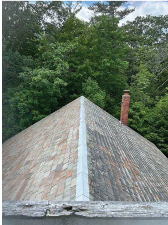
Photo 23 Chimney above roof line
