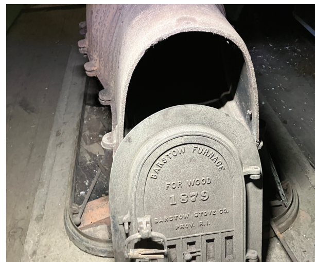
Image B-09: Wood-fired cast-iron furnace, “Barstow Furnace for Wood 1879”
