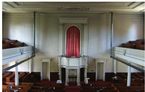
Image A-14: First Parish, Lancaster MA which is heated today via wood fired stove pipes
