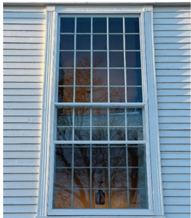
Image A-30: An example of a recently restored window with new storm window
