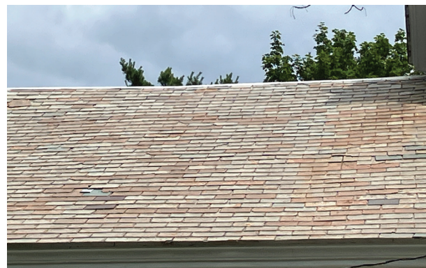
Image A-03: Overall view of south roof plane
