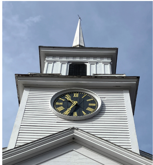
Image A-31: The existing clock faces restored in 2008 remain in good condition
