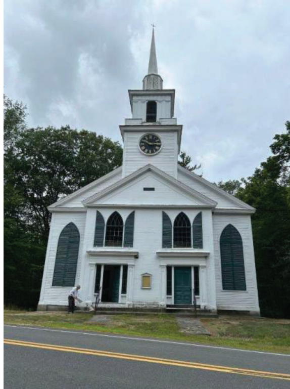
Photo 1 East elevation of the church
