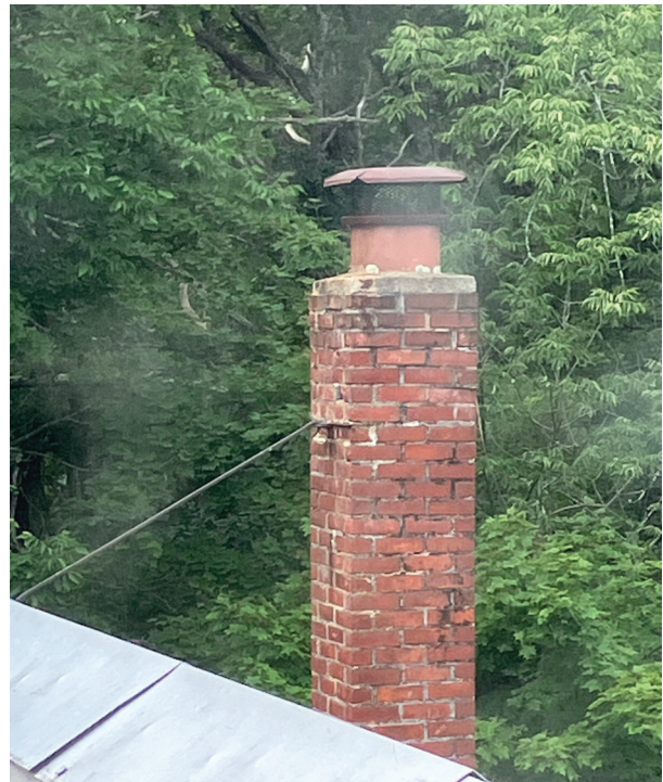
Image A-13: View of existing chimney on the north roof plane
