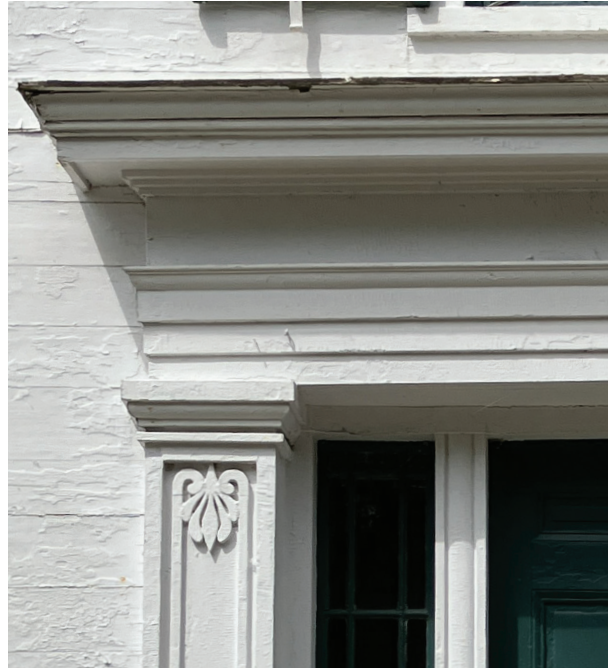
Image A-17: Detail view of entablature corner
