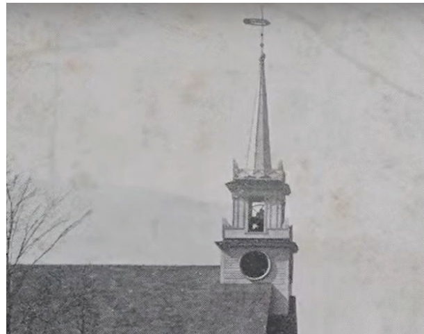
Image A-10: Historic photo shows original steeple and balustrade at belfry roof. Today's steeple is a fiberglass replacement and the belfry balustrade is gone.
