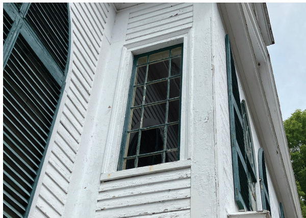
Image A-28: Windows at the return walls of the entry pavilion are wood casement type
