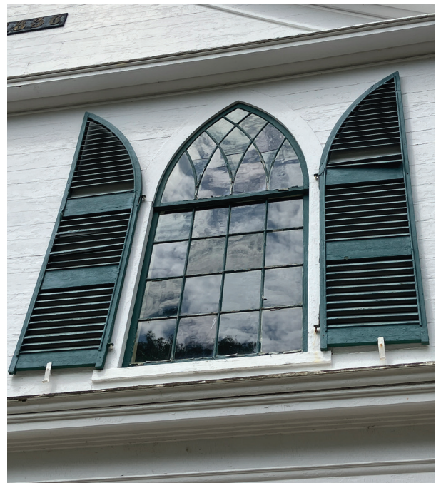
Image A-26: At the east elevation, windows are fixed sash with gothic transom above
