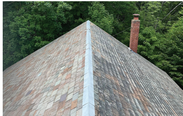
Image A-01: Overall view of roof. Note the wear difference between the north and south roof planes.
