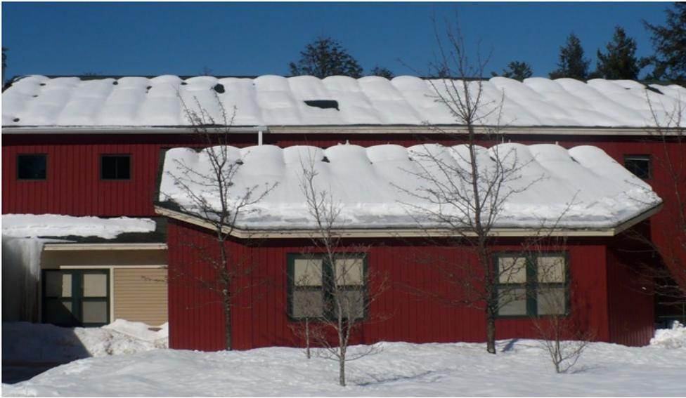
JK has been in touch with Chip Greenberg of Greenberg Associates, the architects for the school. Composite panels called Tectum III (R25) were used with no obvious provisions for air sealing. The energy audit performed by Keith Abbott in 2010 verifies this. Chip said the panels are guaranteed for 15 years, but there is no mention in the Tectum insulation guide for air sealing this product. JK has requested a sample of the panel from Tectum.
